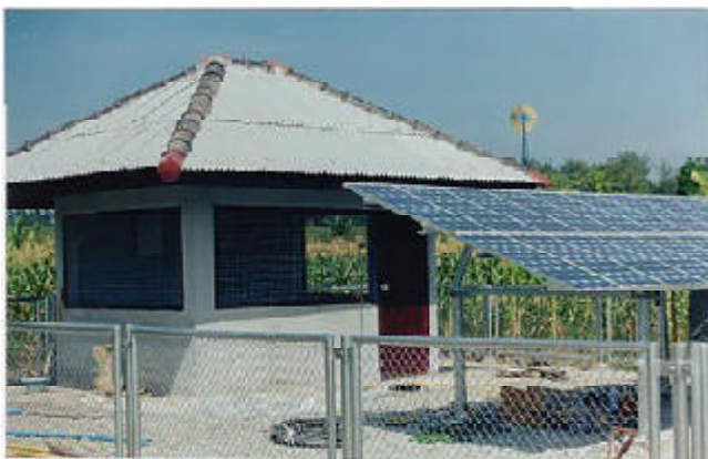
A battery re-charging station in Thailand powered by solar photovoltaic panels.
